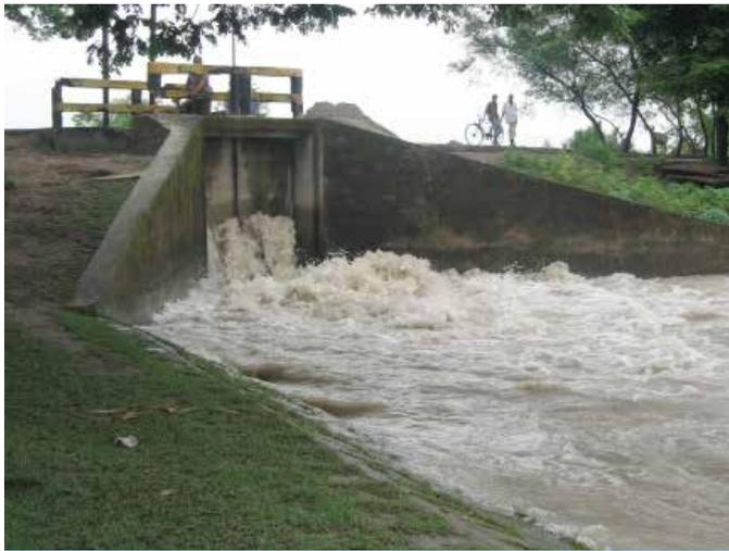
Sluice gate in a polder embankment letting water into the khal for irrigation
