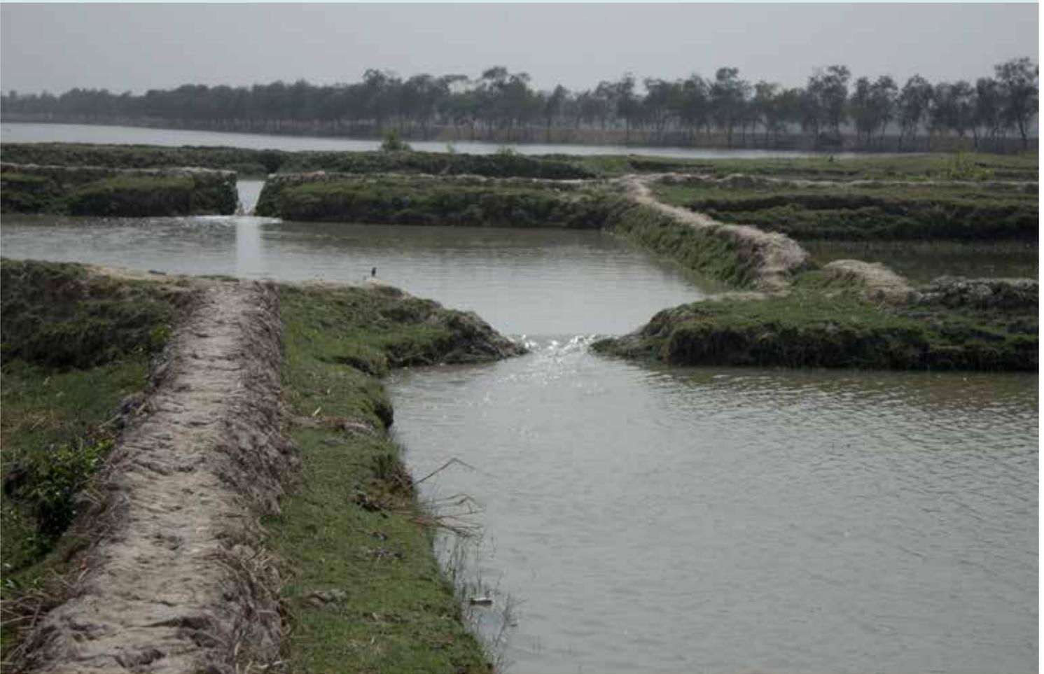
Poor maintenance and informal water intake pipes result in damaged embankments, roads and severe flooding.
