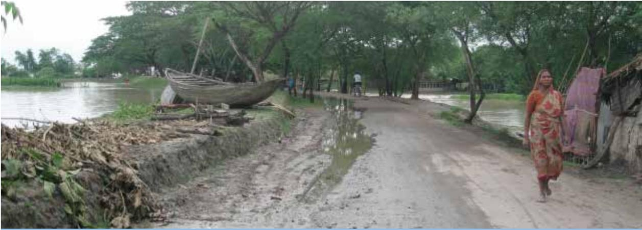
Polder embankment protecting the lands inside the polder (right) from flooding by the river at high tide (left).
