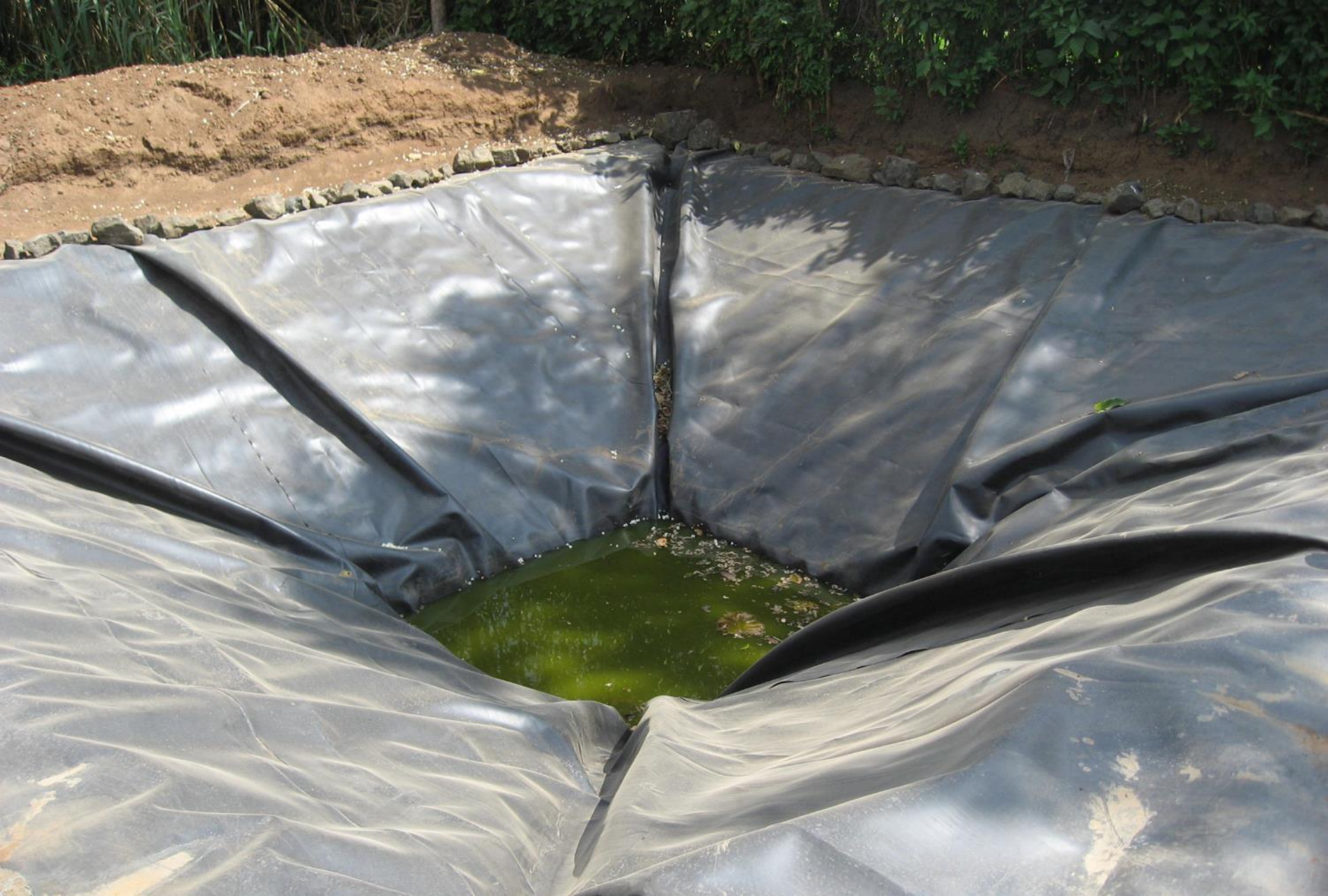
Water harvesting pond with geomembrane – the pond is dug to collect water to irrigate vegetables and fruit trees during dry periods.
