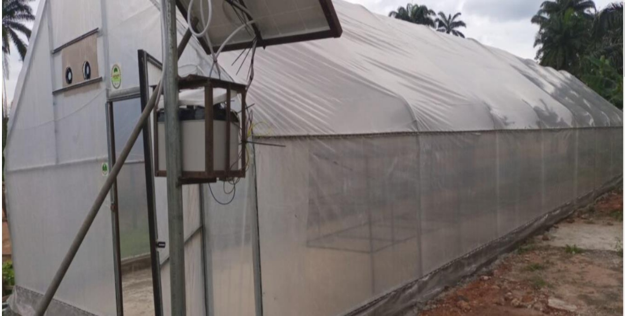
Figure 13:GREEN-HOUSE SOLAR DRYER
