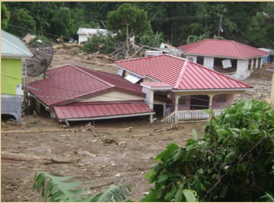
Landslide in Fond St. Jacques, Soufriere
