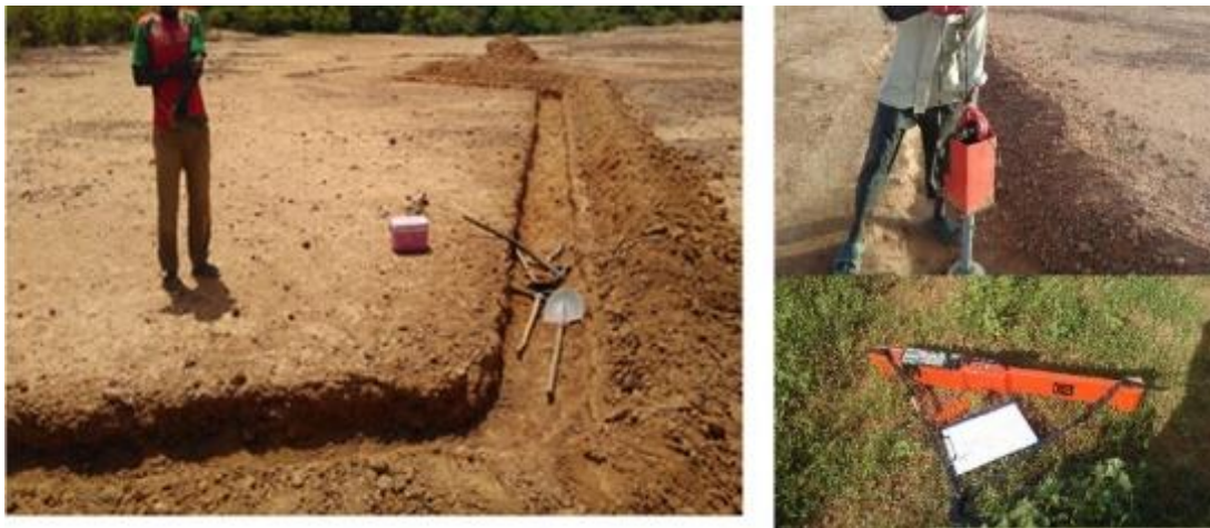
Fig5. Bench terracing with impluvium (upstream), ditch and small land mound. Hydrological measures using neutron probe and water conductivity apparatus.
