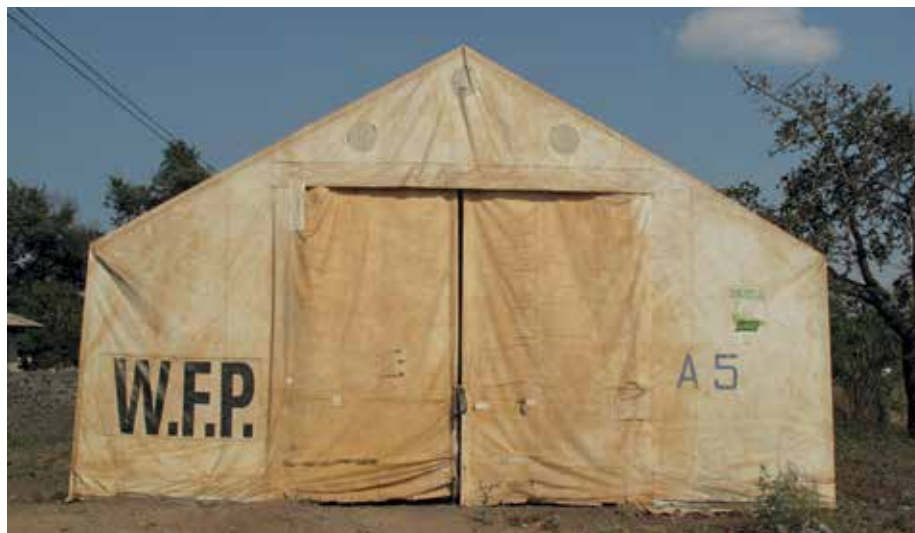
The World Food Programme (WFP) is a major buyer of quality maize in East Africa. It installed this temporary warehouse for the Kware Savings and Credit Cooperative Organisation.
