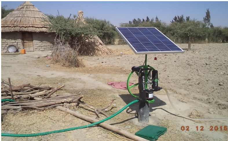
Picture 1: Piloted solar water pumps.
