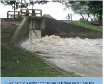
Sluice gate in a polder embankment letting water into the khal for irrigation
