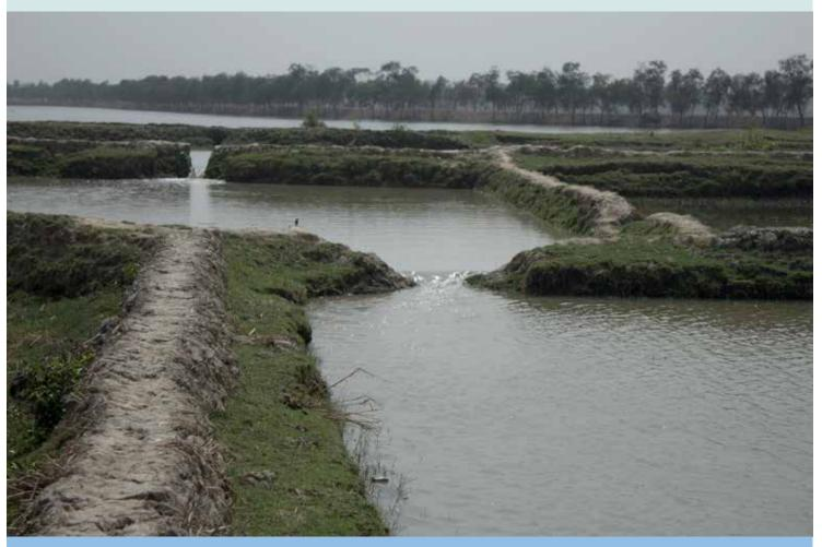
Poor maintenance and informal water intake pipes result in damaged embankments, roads and severe flooding.
