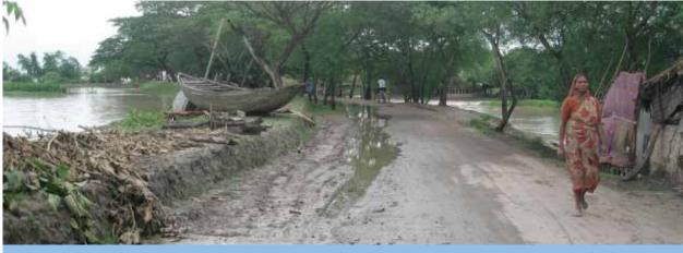
Polder embankment protecting the lands inside the polder (right) from flooding by the river at high tide (left).
