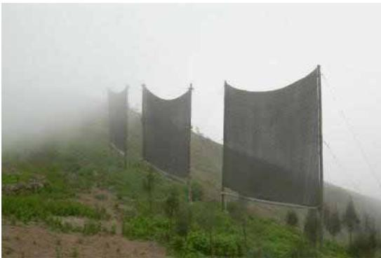
Figure 14 Fog collectors (Source: climatetechwiki.org 2016)
