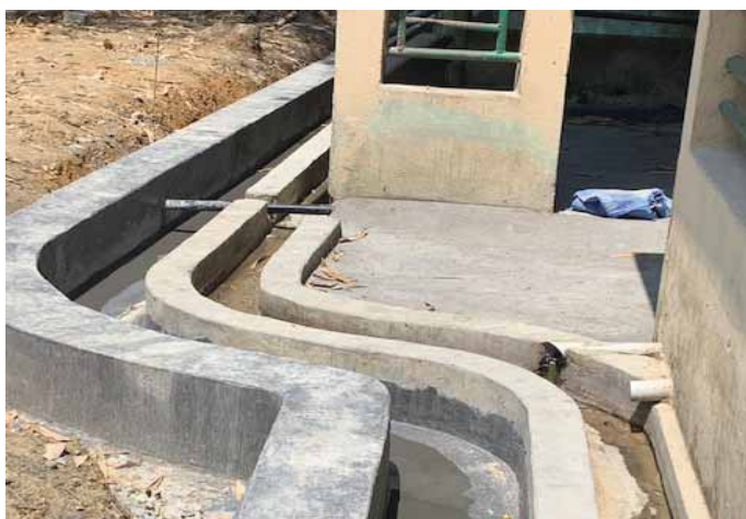
Drainage system in a pig sty
