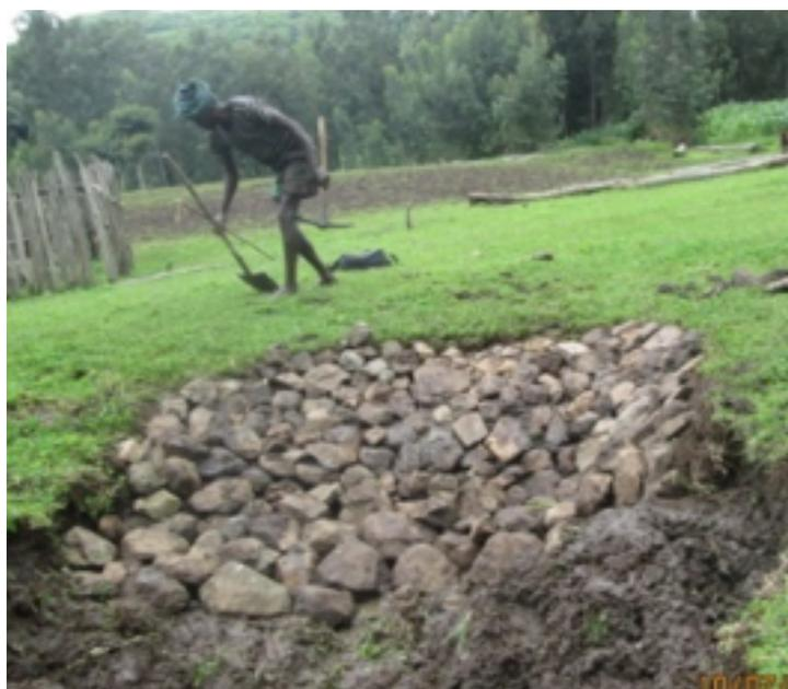
PICTURE 2: GULLY HEAD TREATMENT USING STONES OF DIFFERENT DIAMETERS (PHOTO: MESERET B. ADDISIE)
