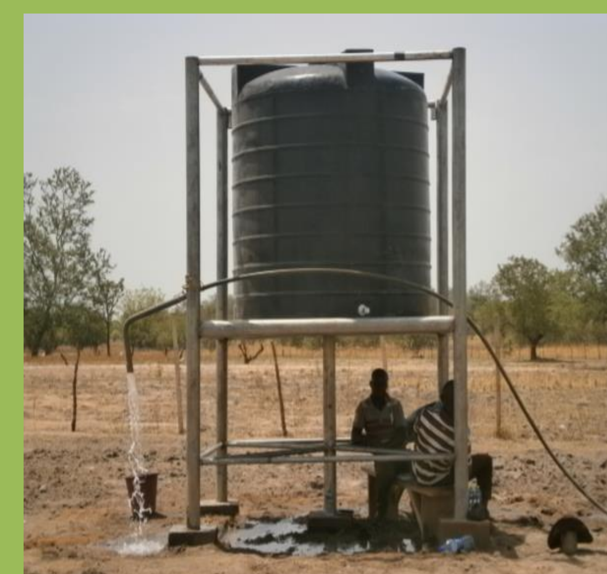
Poly tank as temporary storage for water pumped from Bhungroo. Photo credit: Paa Kofi Osei-Owusu
