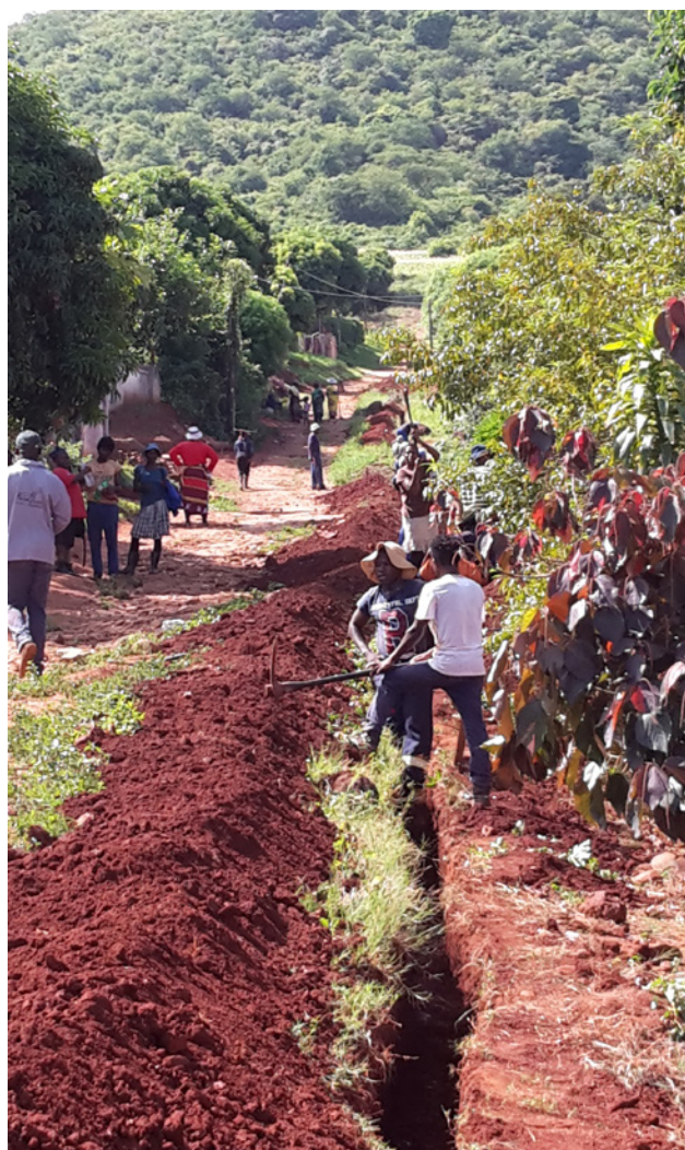
Figure 8. Semiskilled workers digging a trench in Maswie section of Tshakhuma.
