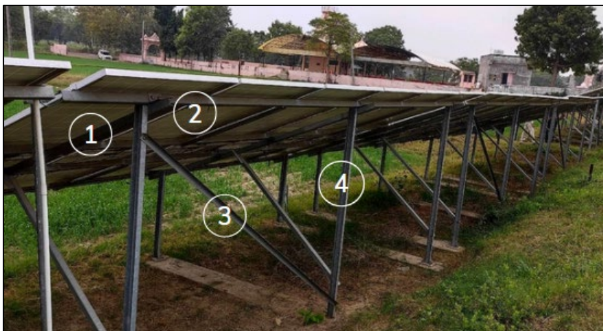
Figure 13. Module mounting structure with different components: (1) RAFTER; (2) PURLIN; (3) BRACING; (4) LEG photo: GERMI
