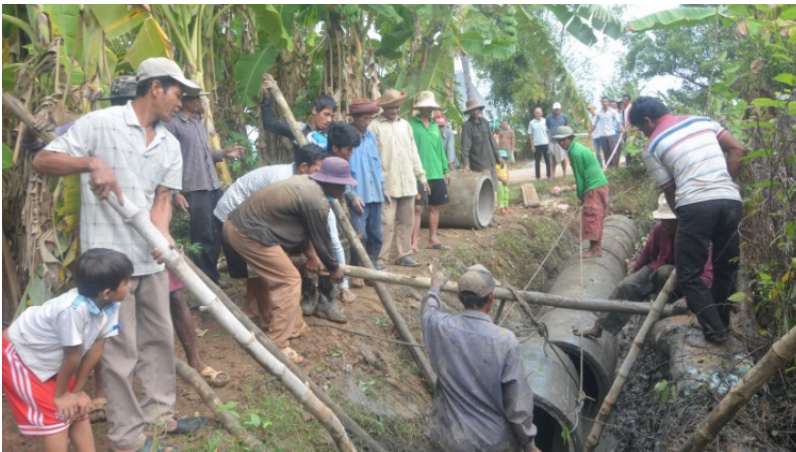
Figure 7. Villagers in Rohal Soung are building an irrigation canal
