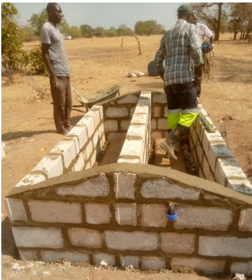
Figure 9. Construction of the water trough in Hanzila community (photo: Miyoba 2025)
