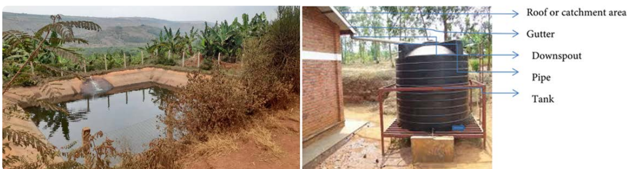
Figure 5: Water harvesting from lake (left) and from rain (right) to the reservoir
