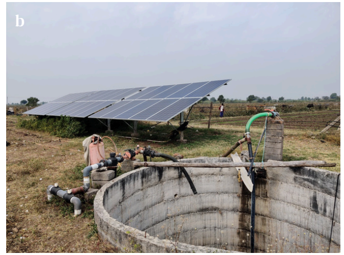
Figure 3. Measuring water application in (a) diesel and solar farmer plots in Bangladesh and (b) flow meter installed at farmers well in India. (Photo: IWMI India)
