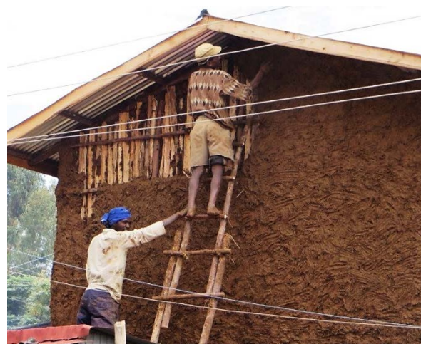
Figure 7: Plastering a new house with a corrugated iron roof in a newly electrified rural community
