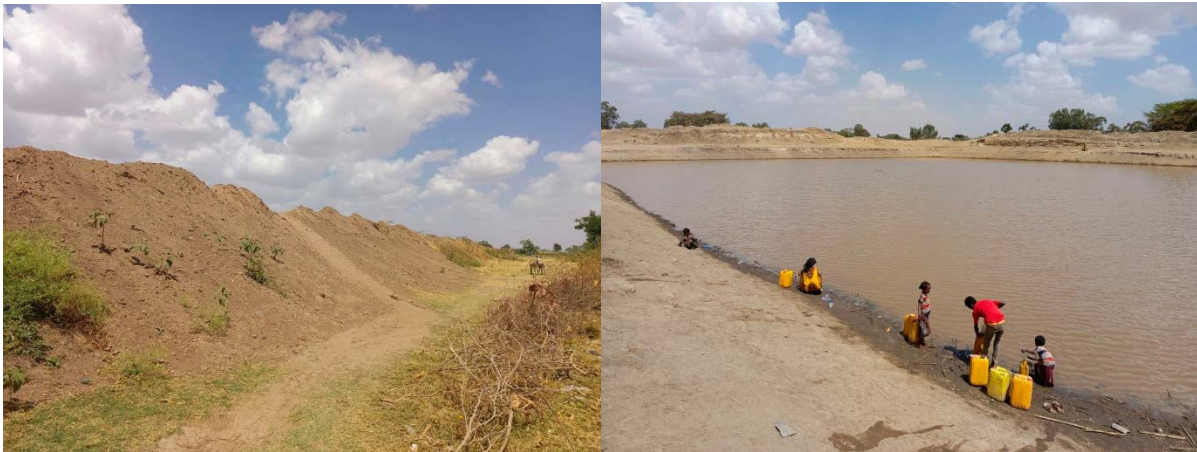
Figure 8. Flood protection dike (left) and flood diversion pond (right) in Wera Dijo woreda.
