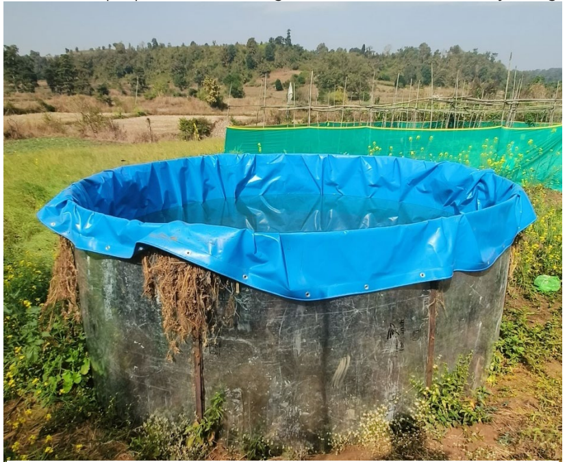
Figure 12 Above ground portable Jal Kund constructed near multilayer plots (Photo: PRADAN)
