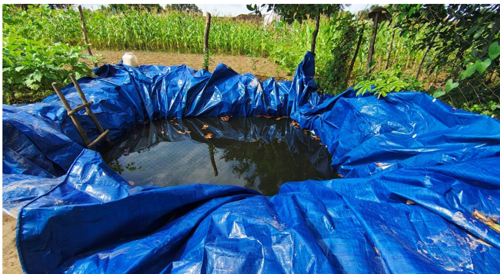
Figure 11 A Jal Kund constructed near multilayer plots (Photo: Green Hub)
