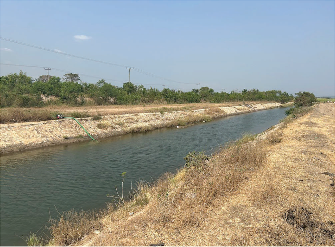
An irrigation canal under the Kpong Irrigation Scheme in Ghana was constructed to supply water to a pumping station for a privately owned banana plantation (photo: IWMI).
