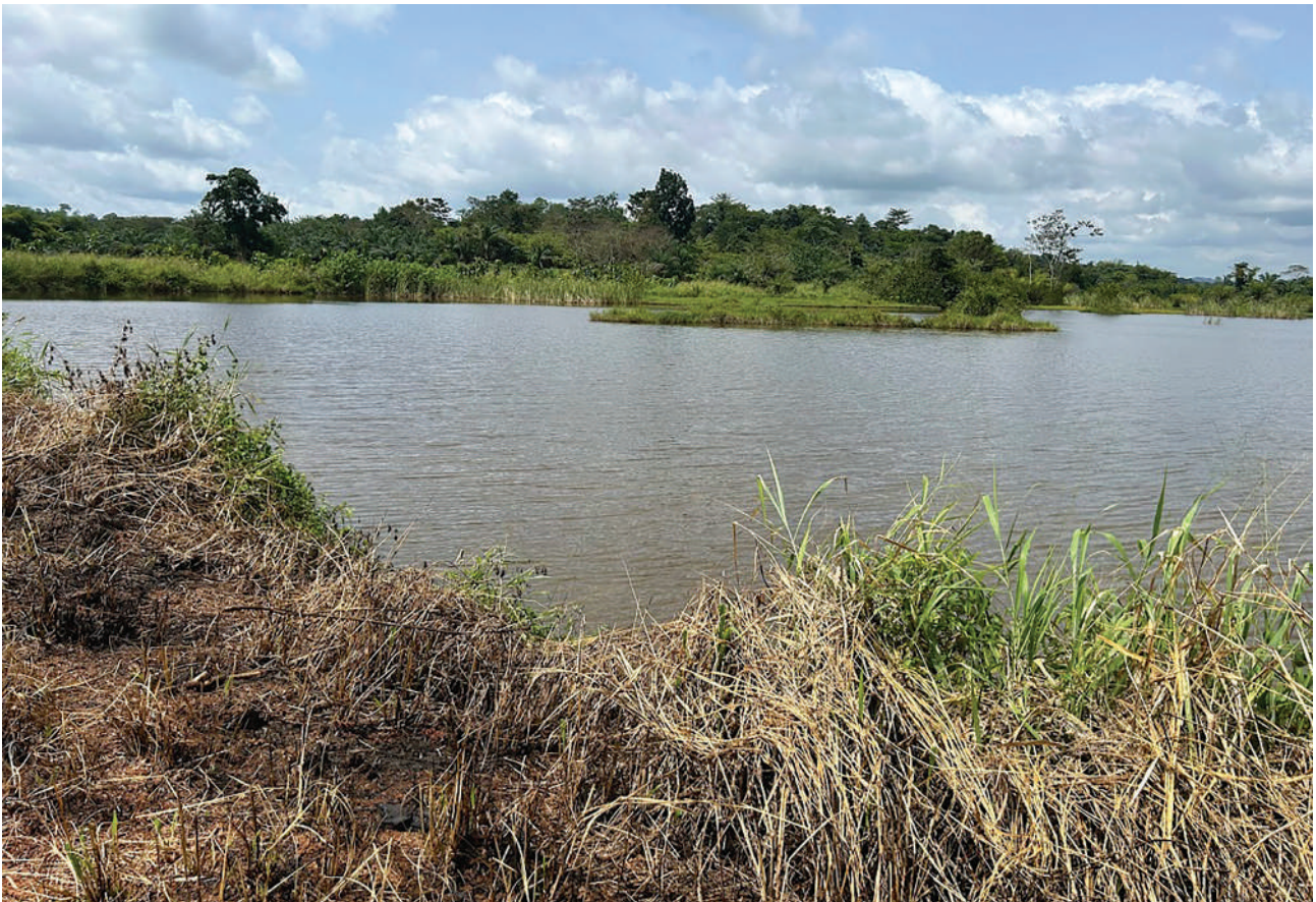
A water harvesting structure located at Potrikrom, Ahafo-Ano South in the Ashanti region of Ghana, serves as a water storage facility under the Inland Valley Irrigation Scheme (photo: IWMI).
