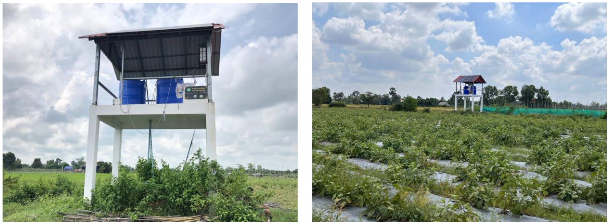
Figure 2. A 1.5-kW community-based SWP system installed by the AIMS project for a vegetable community in Trapeang Ang Village, Kraing Leav Commune, Bati District, Takeo Province (left) and eggplant grown near the SWP system.
