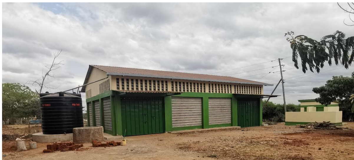
Figure 3.2: Grain store constructed by the Kaka CBO based in Waita Ward, Kitui County
