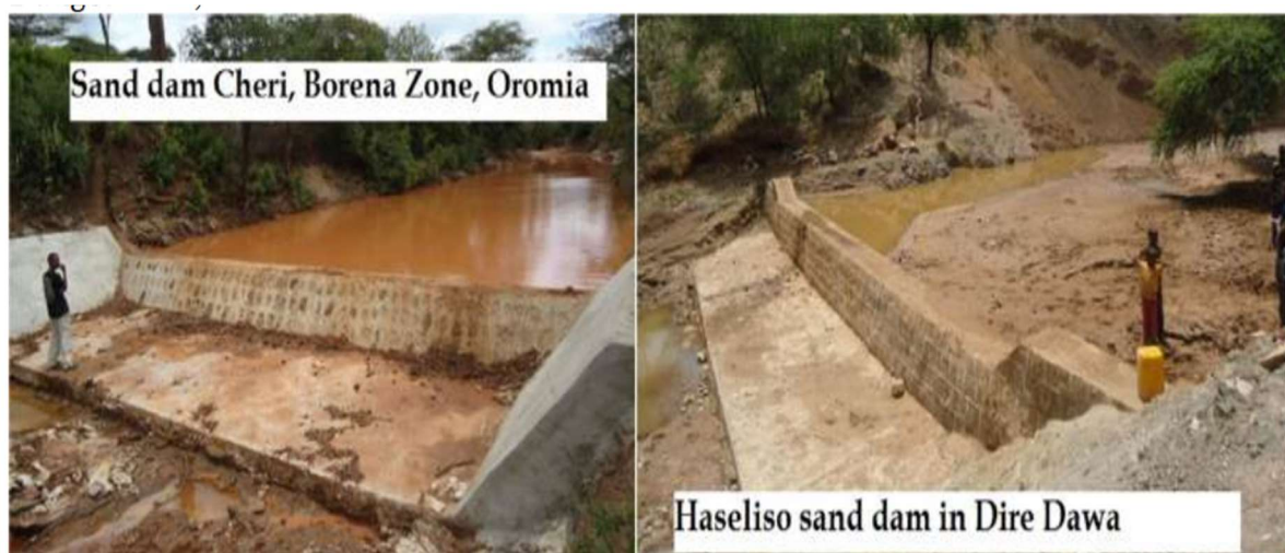
Figure 6: Sand dam/subsurface dam at Borena and Dire Dawa constructed by ERHA
