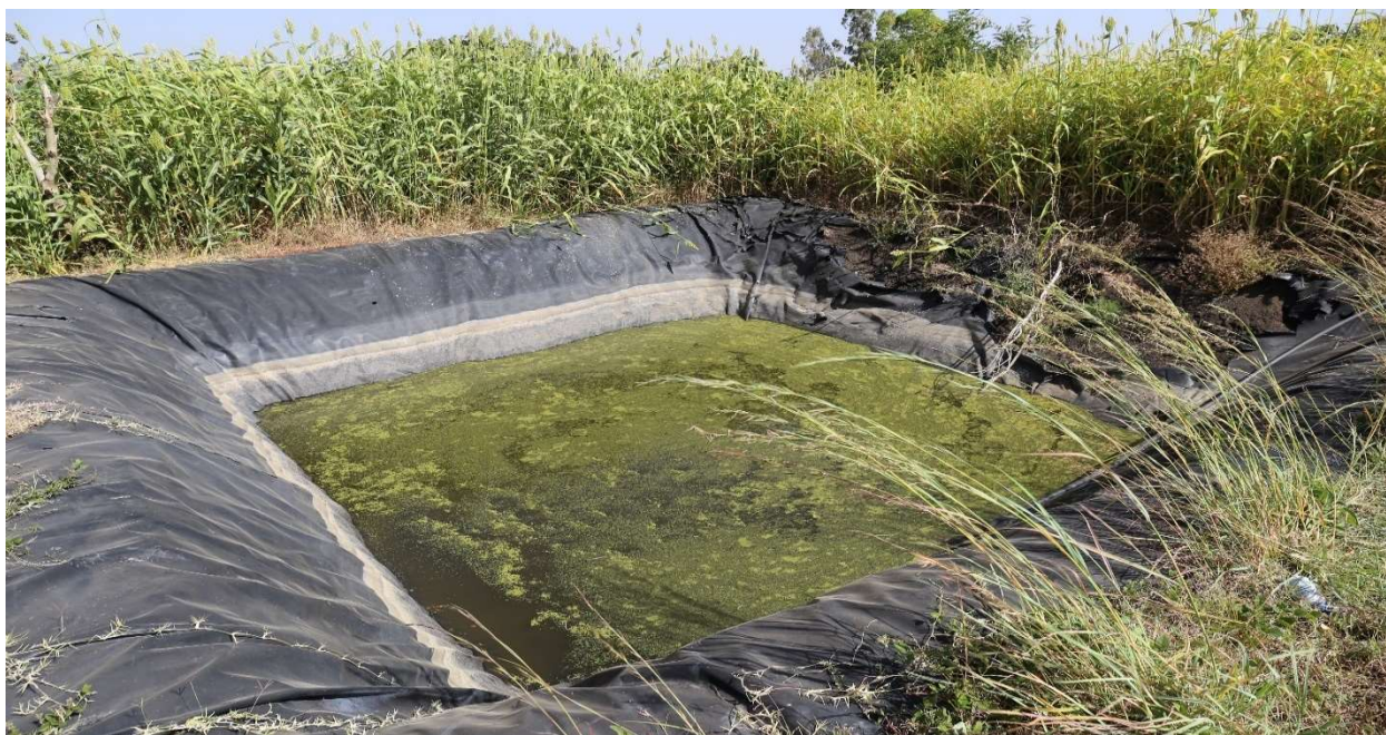
Figure 8: Surface runoff water harvesting through surface pond at Shenkora Woreda
