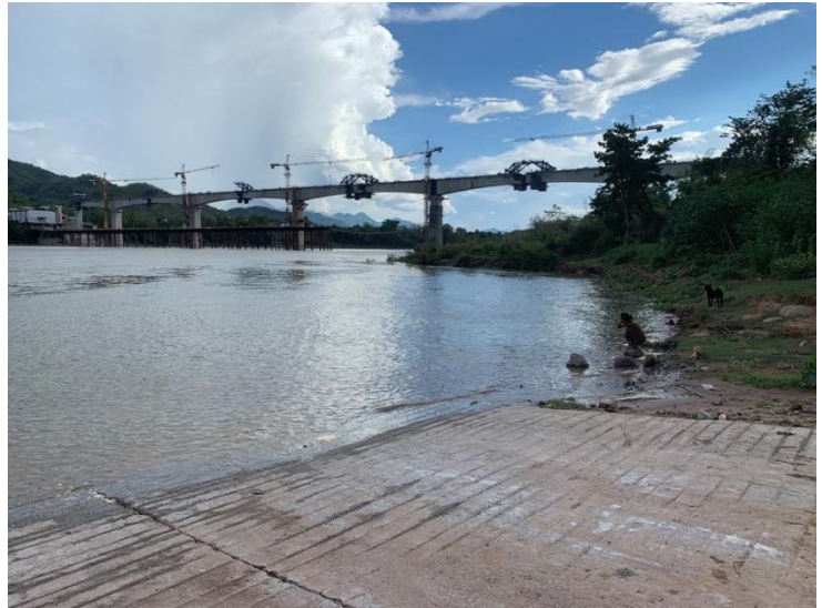
Figure 1 Construction of China-Laos Railway in 2019 (Photo: A.Nicol)
