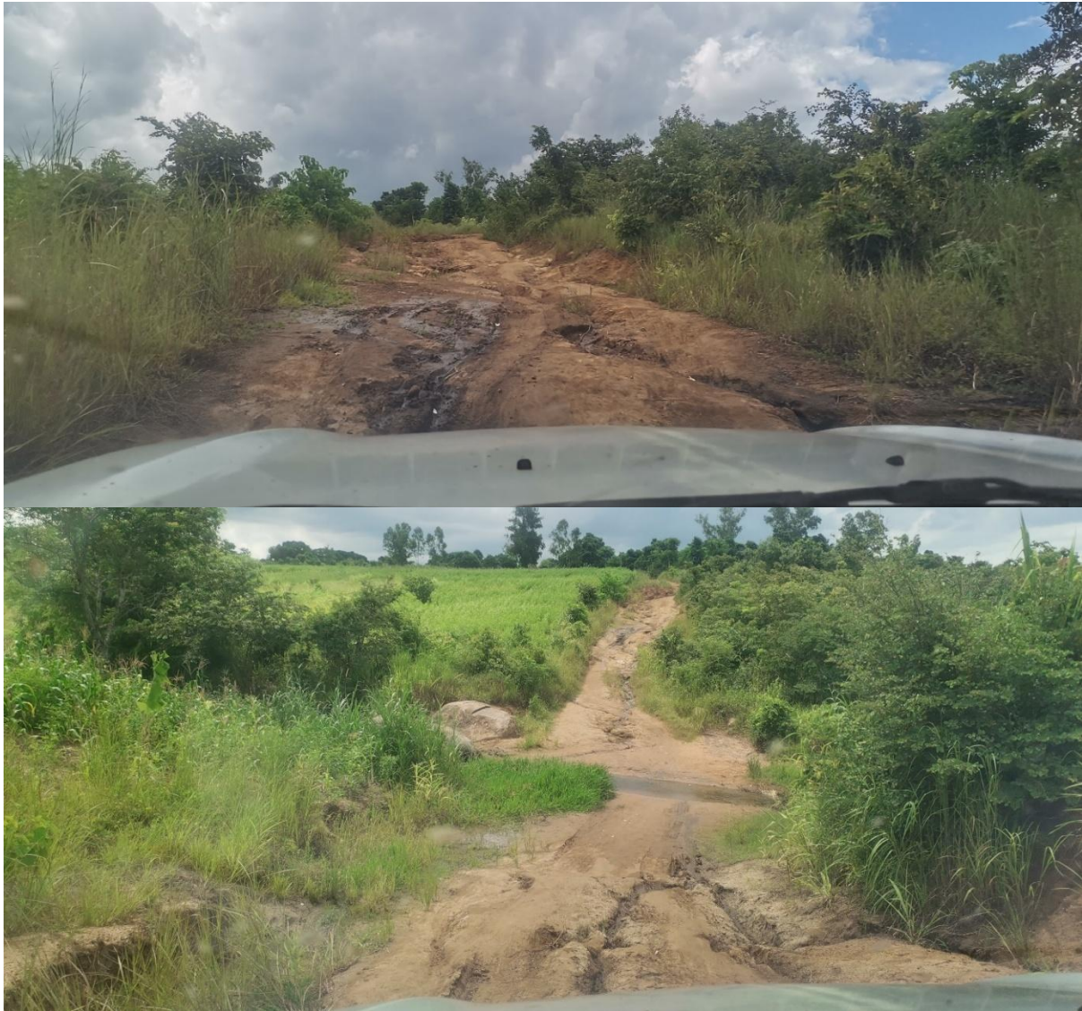
Photo 12. Poor road condition
