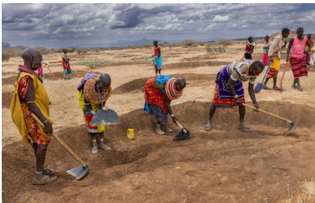
Maasai community digging semi-circular bunds to harvest rainwater and rehabilitate degraded rangeland. Photo by Justdiggit
