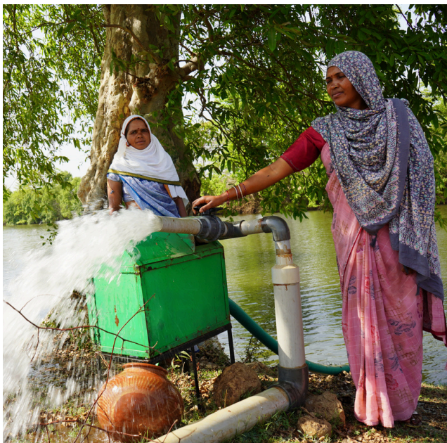
Laxmi Tekab and members of the Bhawarda Water User Association operate a newly installed Solar Irrigation Pump in Bhawarda village, Narayanganj block, Madhya Pradesh. (photo: Tanmoy Bhaduri/IWMI)
