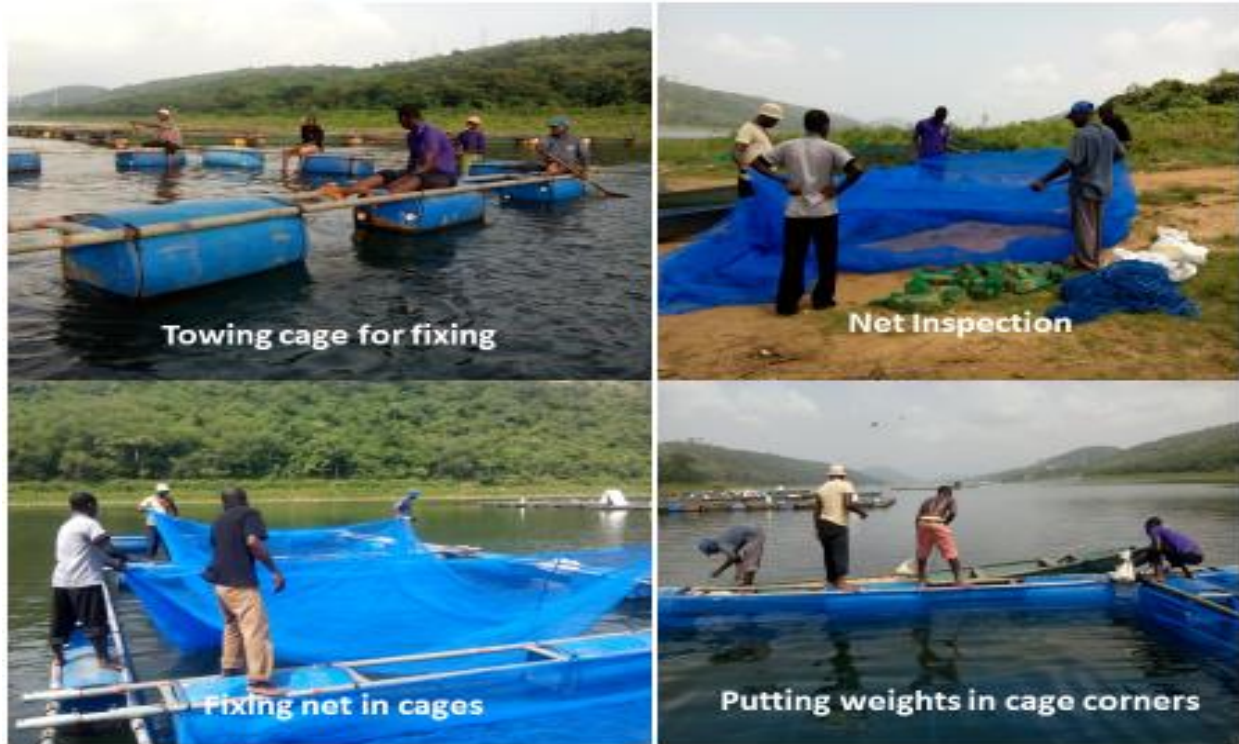
Plate 3-2: How to install your cage on the water (Source: Agyakwah et al., 2018)
