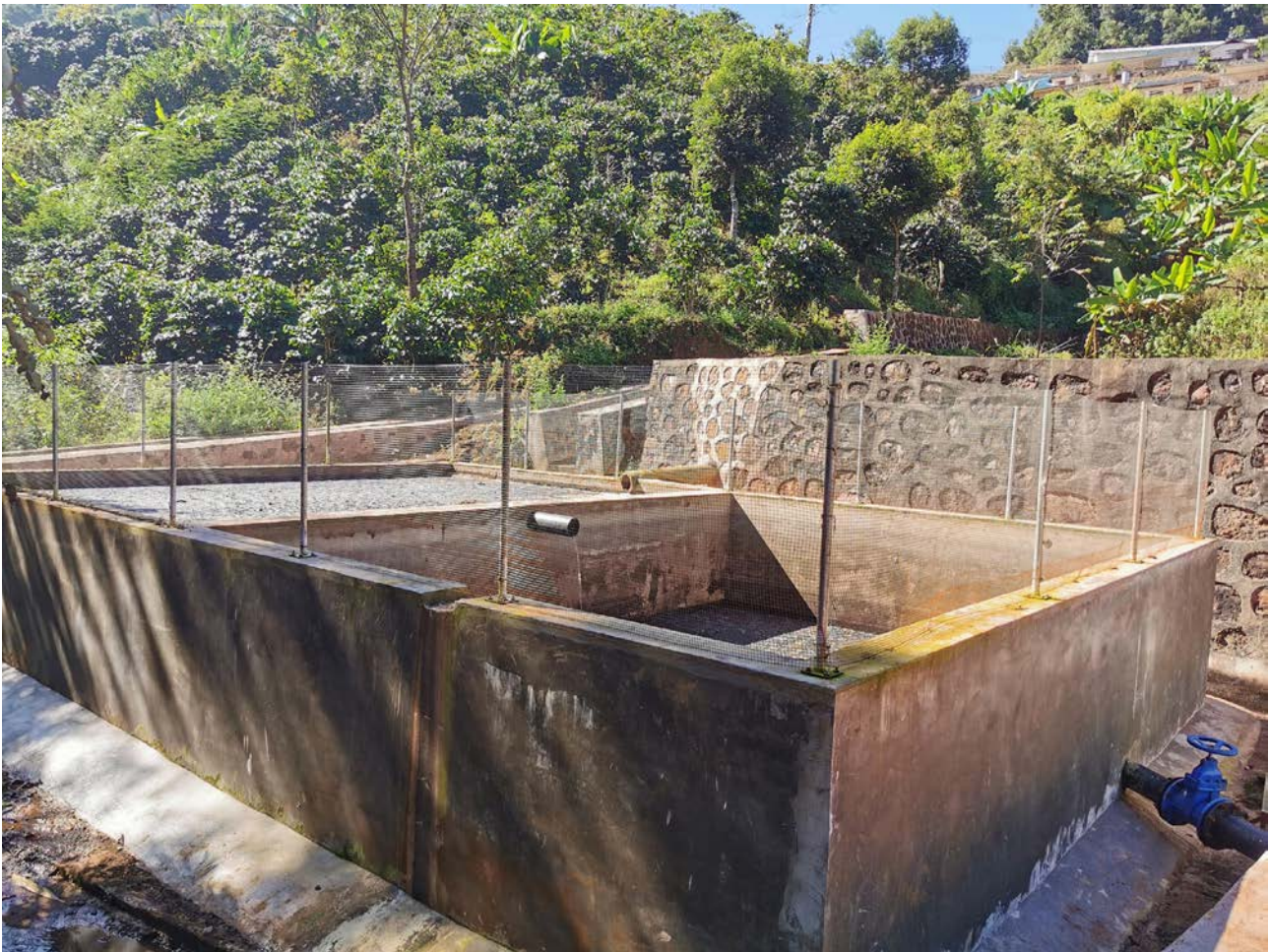
Wastewater treatment tank | Nestlé.
