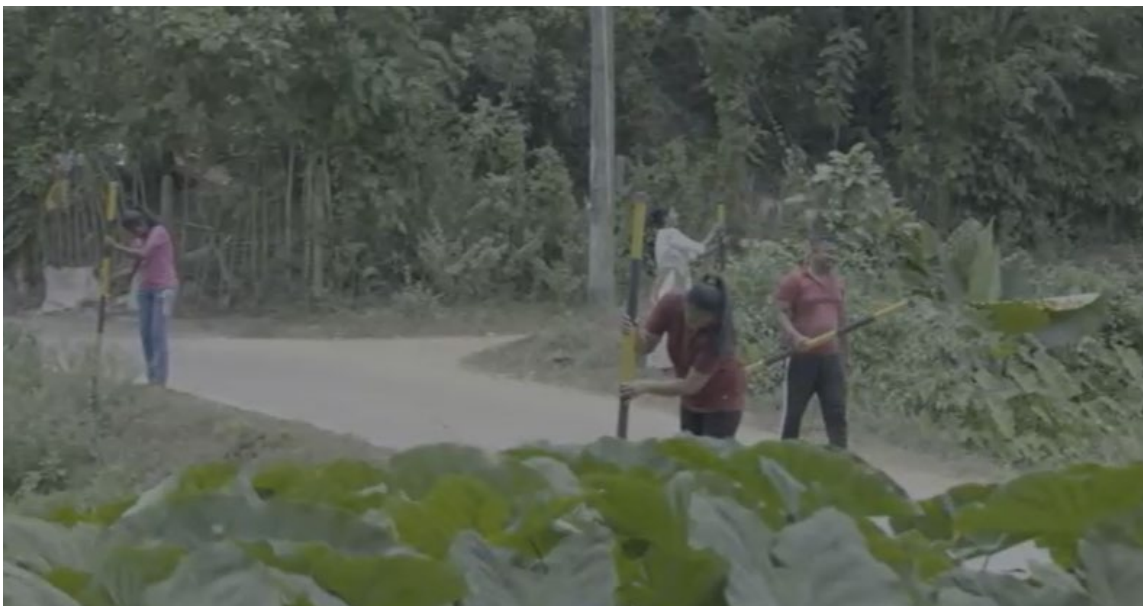
Figure 8: Flood level markers are installed along the road to monitor flood levels and demarcate the road's boundary. (photo: Sakuna/BIZ)
