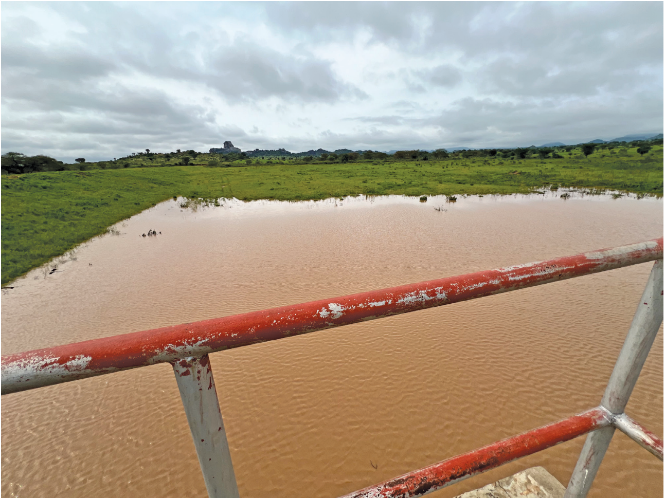
FIGURE 3. Longoromit Dam, Kaabong, Uganda, in July 2024 (Photo: Alan Nicol/IWMI).
