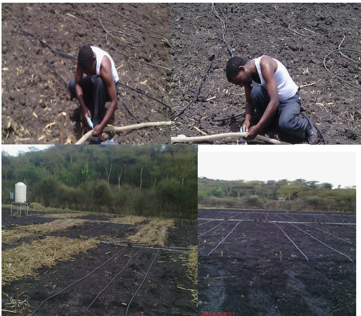
Appendix Figure 1. Drip installation and mulching
