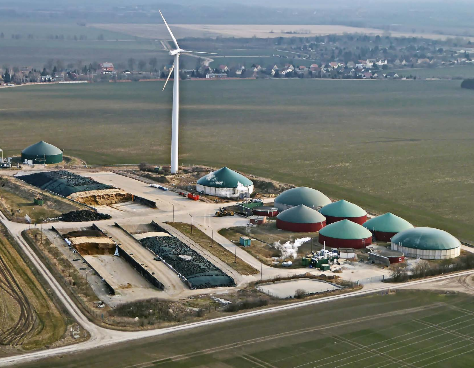
Biogas plant - Westeregeln near Magdeburg, Deutschland. Photography by René
