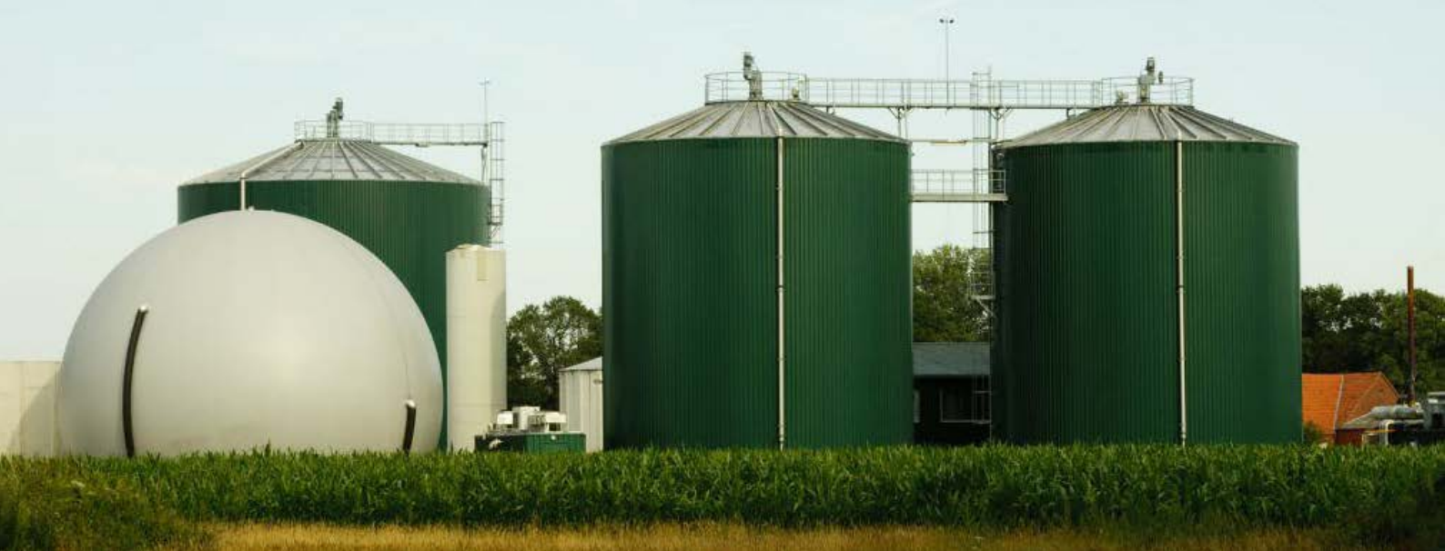
A large biogas plant in North Carolina. Photography by Shaun Edward Lee
