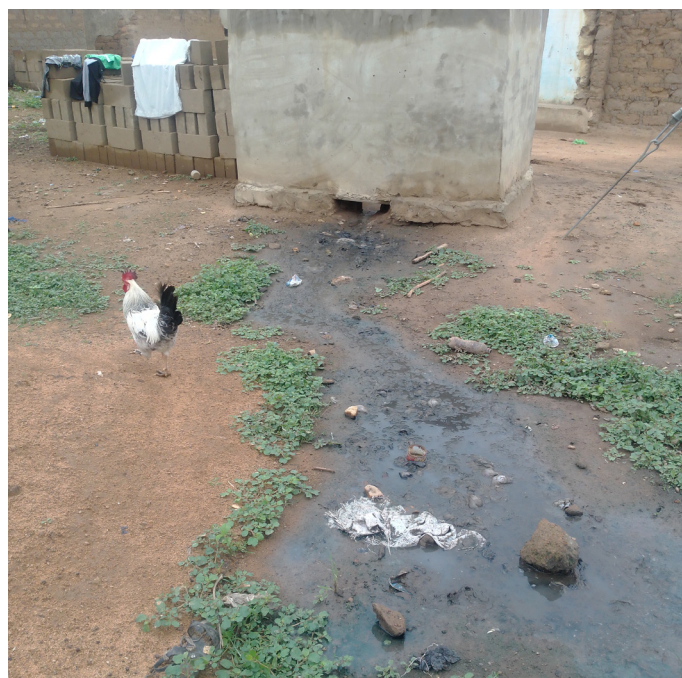
Greywater from bathrooms channeled into the open in Kpong, Ghana (photo: IWMI).
