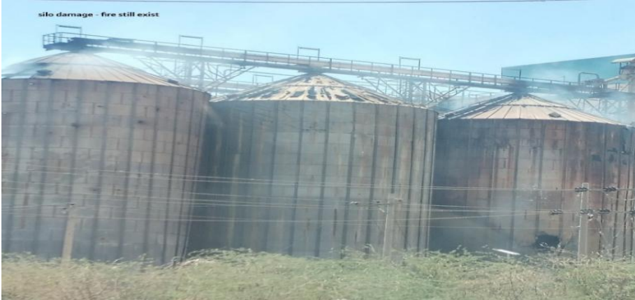
Source: Photo taken by site visit team during field assessment, March 2025.
