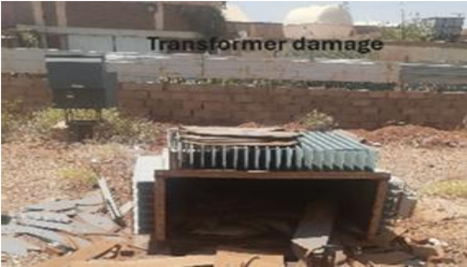
Source: Photo taken by site visit team during field assessment, March 2025.
