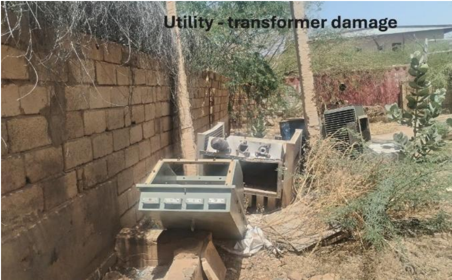
Source: Photo taken by site visit team during field assessment, March 2025.
