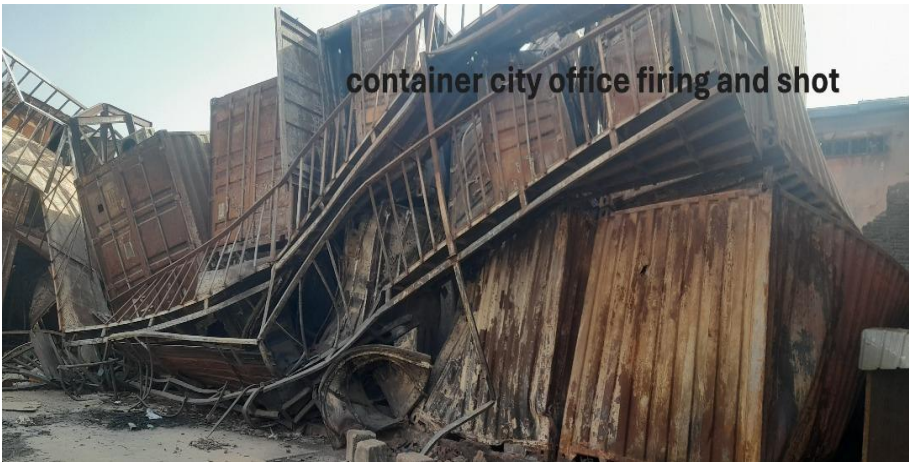
Source: Photo taken by site visit team during field assessment, March 2025.
