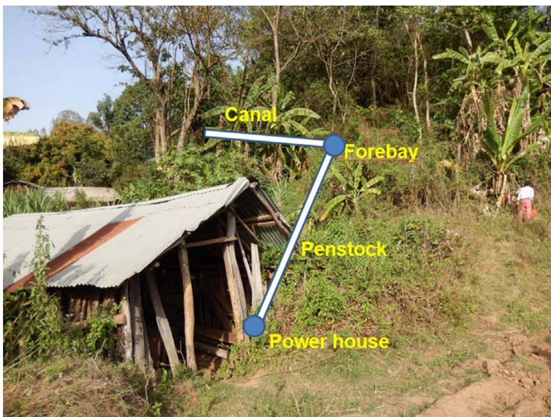
Figure 39. Panoramic view and penstock (and powerhouse) site of the proposed Barudemeti MHP site, Oromia region, Ethiopia.
