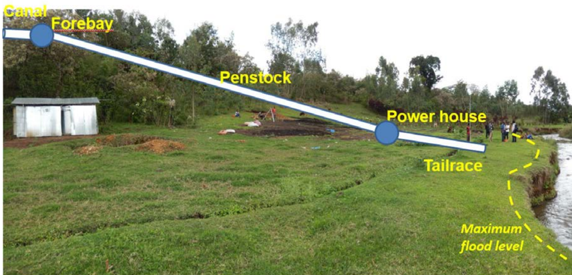
Figure 20. Schematic view (above) and panoramic view and penstock (and powerhouse) site (below) of the proposed Agaro MHP site, Oromia region, Ethiopia.
