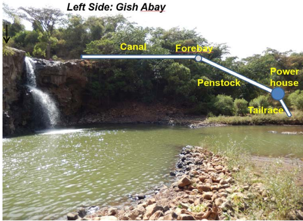
Figure 6. Schematic view (above), right-side option panoramic view (middle), and left-side option panoramic view (below) of Gilgel Abay MHP site, Amhara region, Ethiopia.
