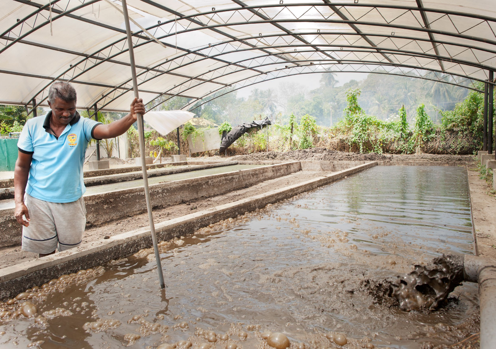
Measuring the fecal sludge (human waste) at Dikowita Bio Gas Unit, Western Province, Sri Lanka. Photography by Hamish John Appleby / IWMI
