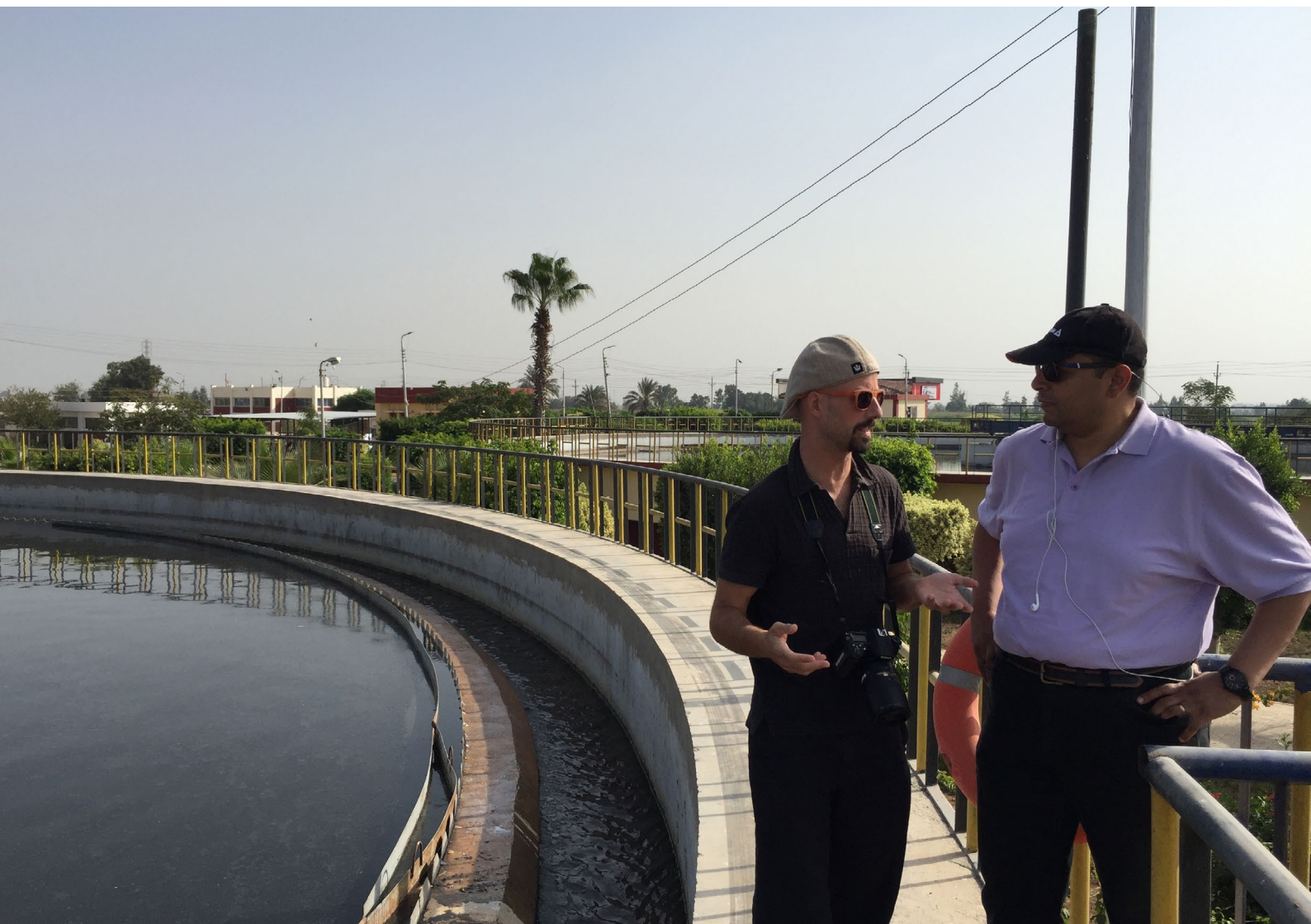
Wastewater treatment plant in Sakha village in Kafr El Sheikh governorate, Egypt. Photography by Gihan Bayoumi / IWMI
