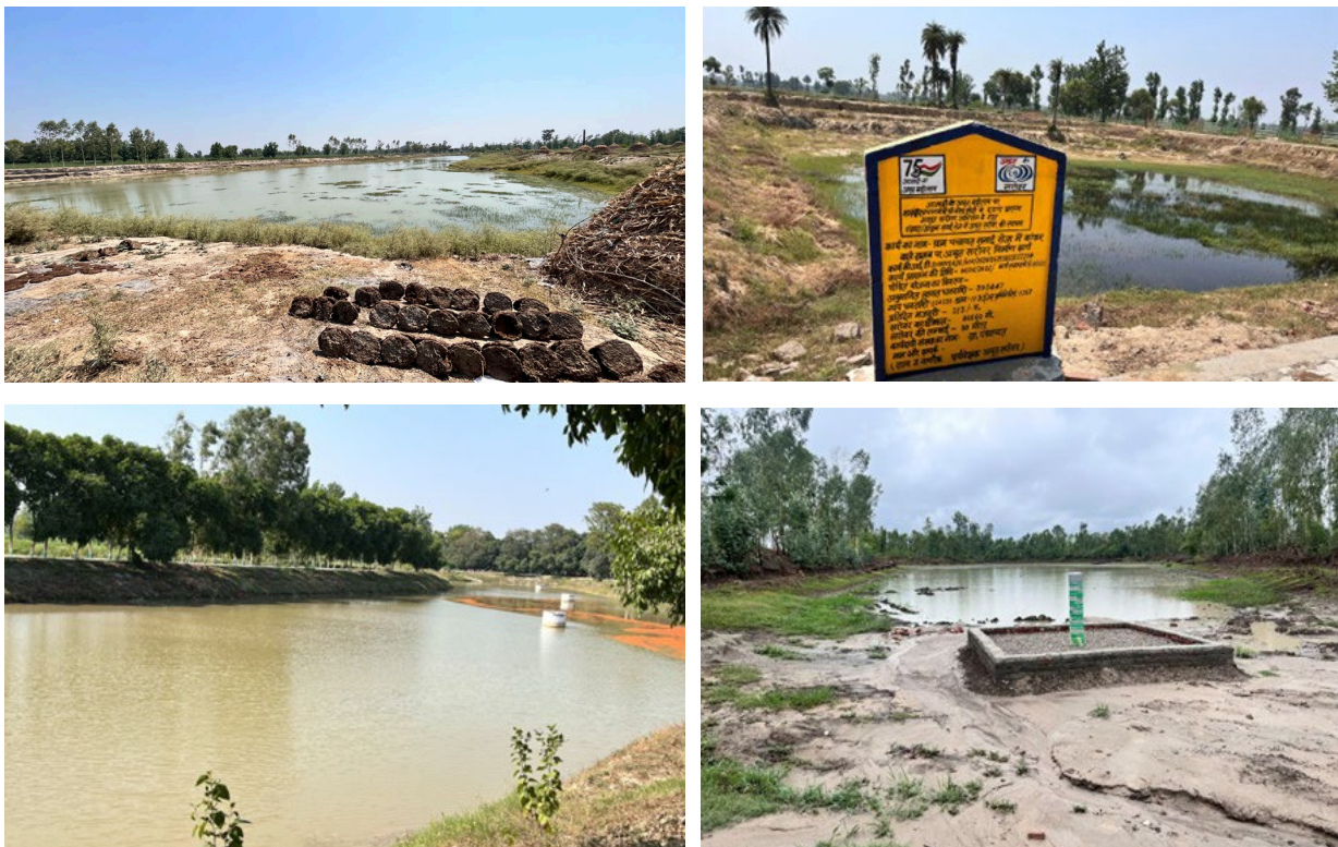
Figure 2. Representative photos of the a) Control pond, b) Repurposed pond, c) Repurposed pond with recharge wells and d) Repurposed pond with recharge pits ( photo: IWMI )
