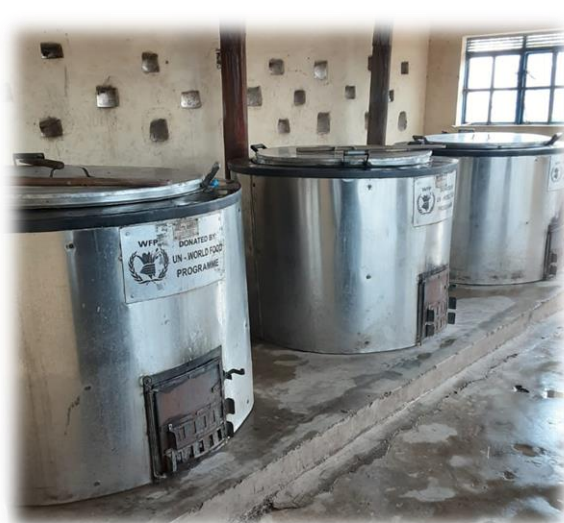
Figure 12: Improved Institutional Firewood Cookstoves in a School in Kalobeyei Integrated Settlement (Photo Credit: SNV EnDEV)
