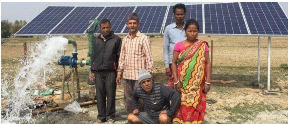
Figure 4. Gham Power has developed an integrated solution called –Yield Improvement in a Box– that provides farmers with reliable irrigation through solar water pumps, easy and affordable financing, and knowledge of modern agricultural practices through personalized agri-advisory. (photo: Gham Power Nepal Private Limited)
