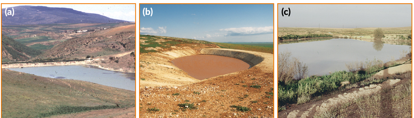
Figure 9. Wadi bed rainwater harvesting reservoirs: (a) A surface reservoir for supplemental irrigation in southern Turkey; (b) An on-farm reservoir in northern Syria; and (c) A surface reservoir with a spillway supporting barley cultivations in the Jordan Badia.
