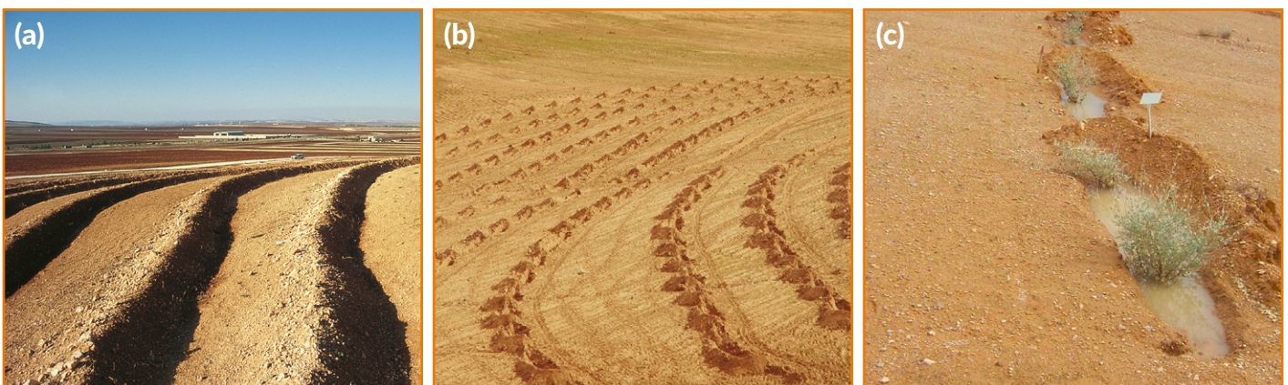
Figure 3. Contour ridges and bunds: (a) Manually constructed contour ridges before planting; (b) Mechanically constructed contour bunds; and (c) Vallerani bunds planted with shrubs in the rangelands of Jordan.
