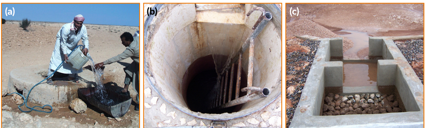
Figure 13. Traditional rainwater harvesting cisterns: (a) An old cistern for human and livestock water consumption in northern Egypt; (b) A traditional cistern renovated for household use in Syria; and (c) A settling basin and gravel filter constructed to clean the runoff water before entering a cistern in Syria.
