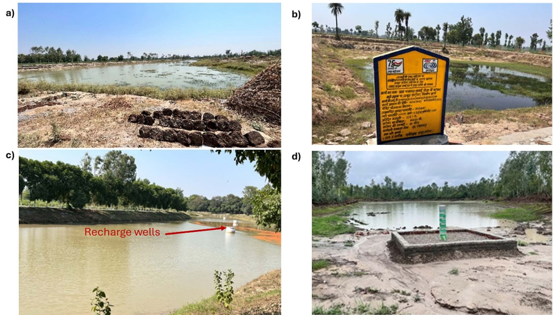
Figure 3. From top left (a) Control ponds (Sanai Roza), (b) Repurposed ponds (Sanai Roza (Amrit Sarovar)), (c) Repurposed ponds with recharge wells (Segankendra). Water enters recharge wells from the top to ensure minimum pond water for other purposes and (d) Repurposed ponds with recharge pits (Changeri).
