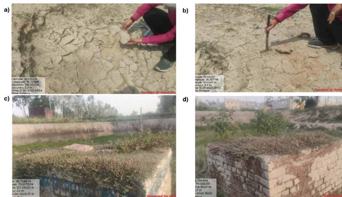
Figure 5. Deposited sediment in pond surface in Imratpur Seondara site (a), (b) and grassy vegetation on recharge wells in site (c) Tumdiya and (d) Daniya Sankarpur.
