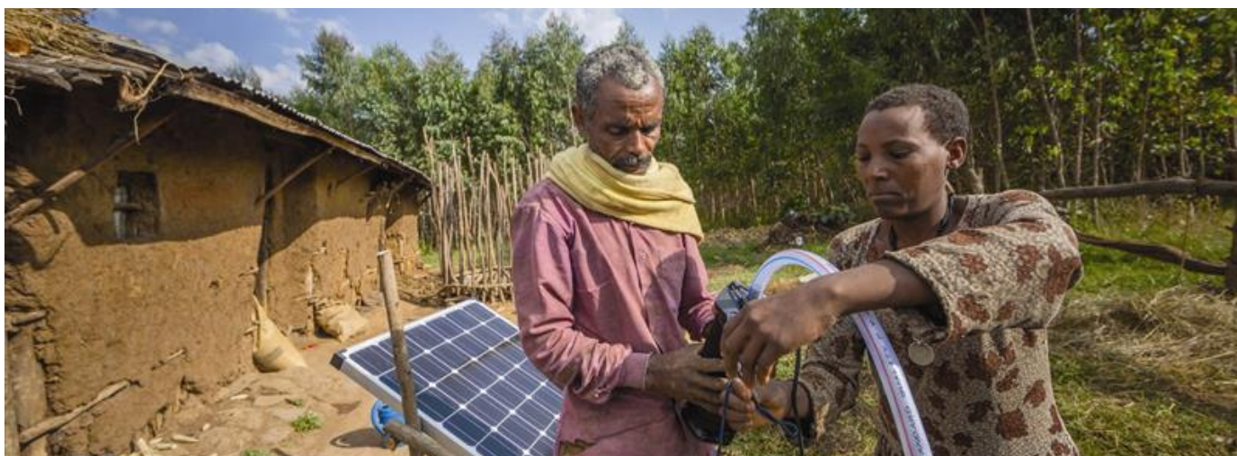
Installing a solar-powered irrigation system in Danghesta, Amhara region of Ethiopia (Photo: Mulugeta Ayene/WLE CGIAR)
